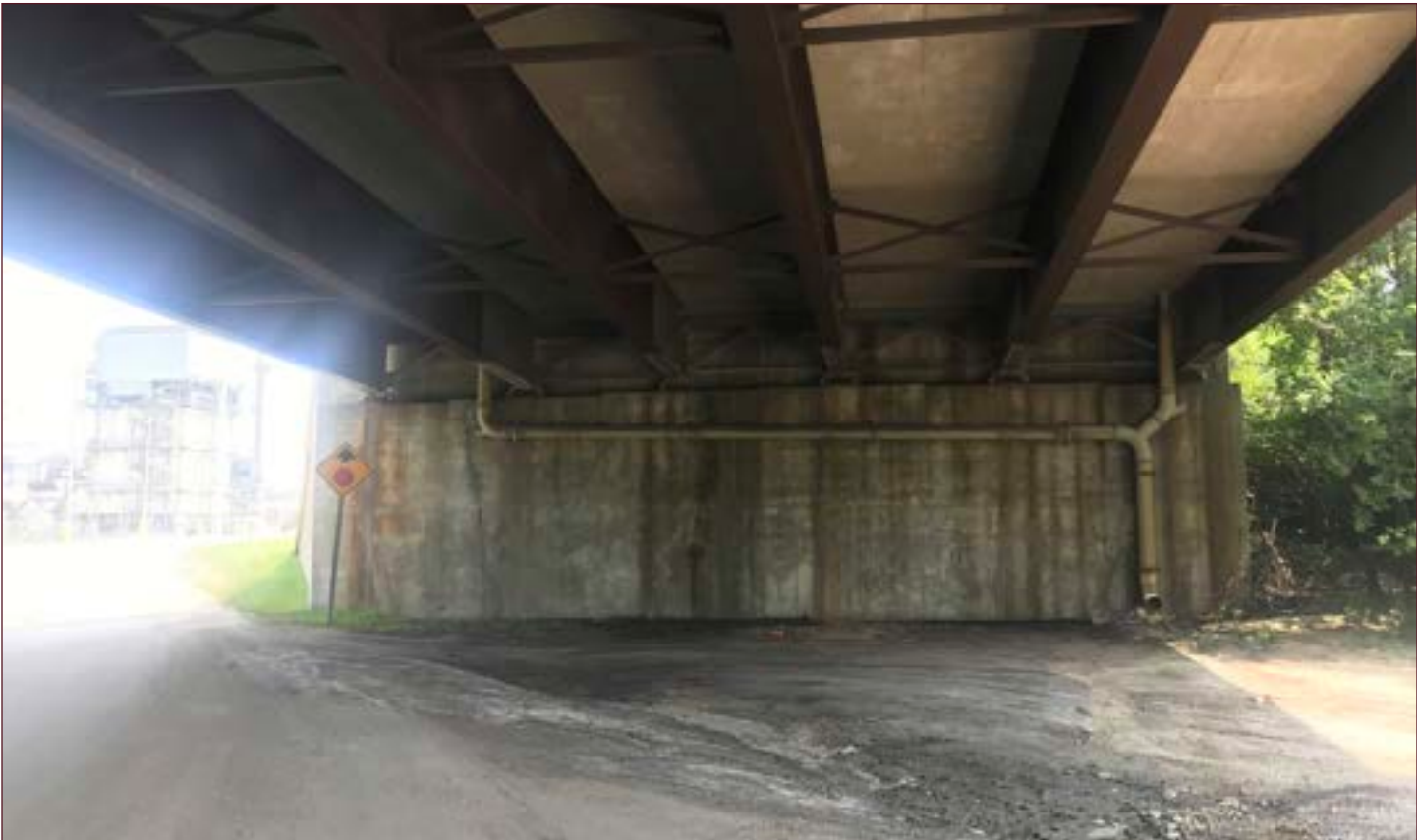
Looking east - headwall
